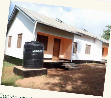
Constructed with support from TAG, teacher housing at Engusero is now complete.
