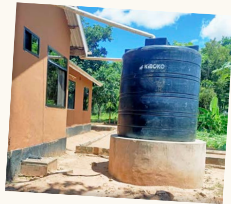
A rainwater harvesting tank was repaired, which now makes it a reliable source to access water in Milola.
