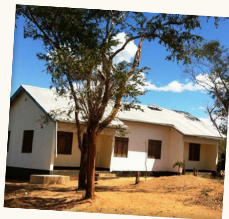
Teacher housing constructed at Ngwenya Primary School supports teacher retention.
