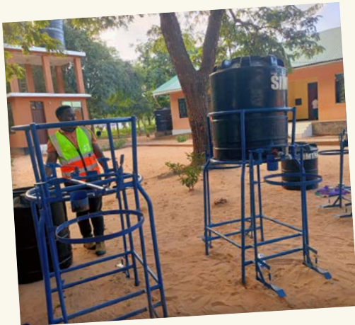
Dennis Meela (UDSM) repairs handwashing stations at Milola Secondary School.
